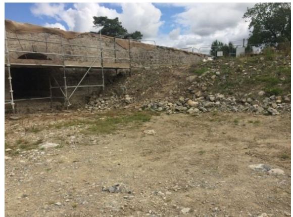
Re-pointing and patch repair well progressed on downstream face of bridge.
