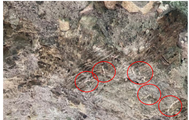
close-up of repair of cracks in wicker
