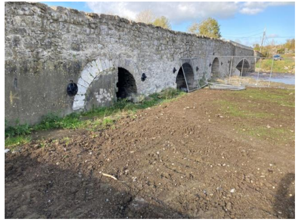
General view of upstream face of the bridge. For structural reasons the existing part infilling of arch A was not undone but the 20 th century cement based plaster was carefully removed from the voussoirs to allow appreciation of the original arch and the rhythm of the whole composition.
