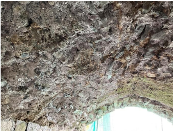
View looking downstream
