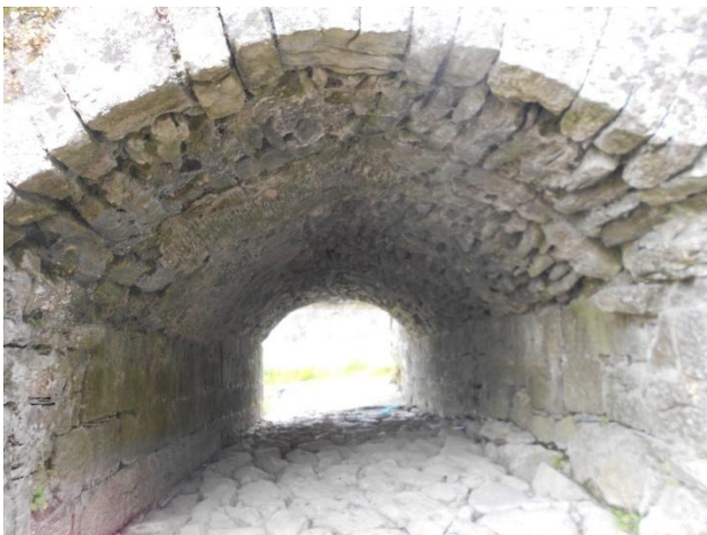
View looking upstream
