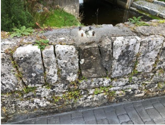
14 Sept 2020. Damaged stone and redundant light fixing. Tapping of wall to test for soundness revealed several loose stones
