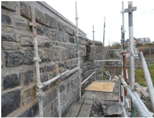
January 2020, stone cladding on the sides of the new bridge is close to completion Upstream side looking north
