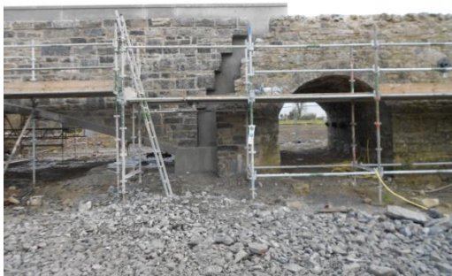
View of break between new bridge span and arch D, downstream side.
