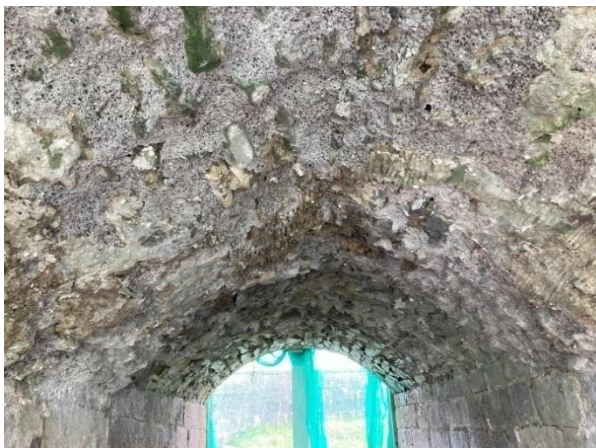
Looking upstream - views of general consolidation of stonework
