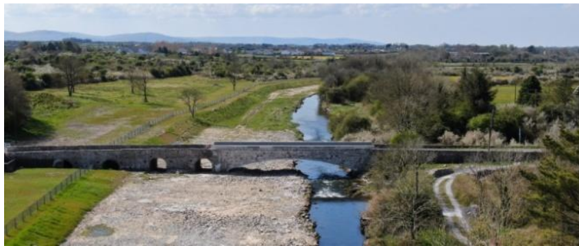
Aerial view of Dunkellin bridge following completion of works Photographs courtesy of Galway County Council
