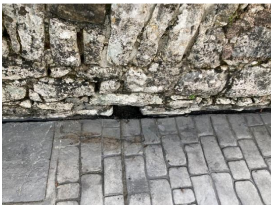
View of joint at an outlet
