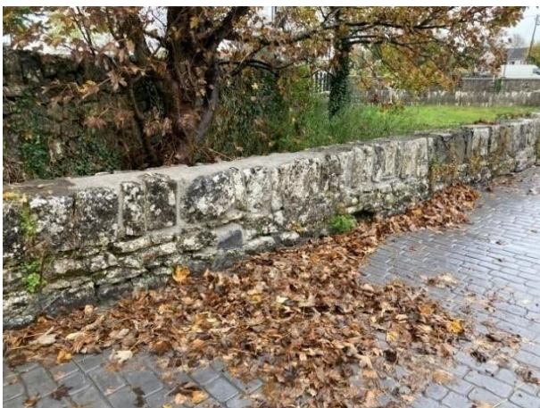
Repaired section of wall, Oct 2020, upstream side, north end
