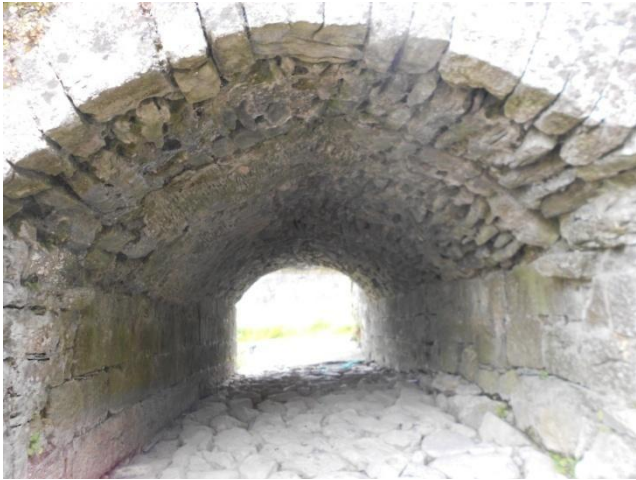
Arch A, View looking upstream Photographs May 2020 prior to works
