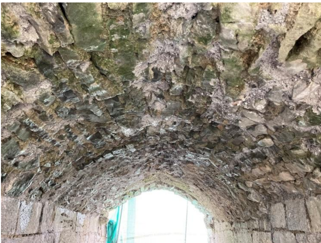
General view looking downstream
