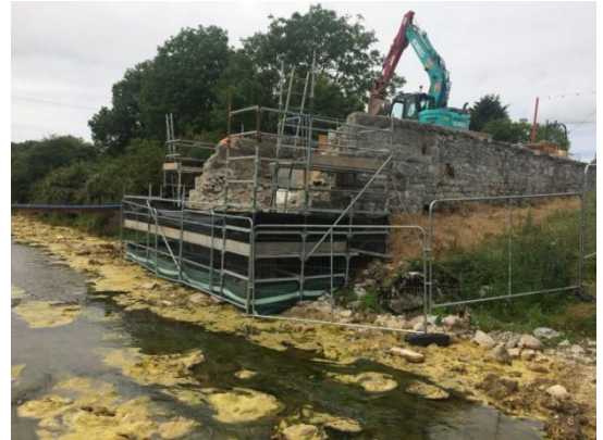
July 2019, preparatory work underway for new concrete support at northern abutment.
