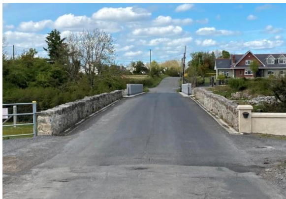
Views taken in May 2021. General view looking north.
