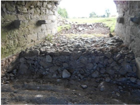
Photographs taken 10 August 2018 Accumulated material on arch floor being removed. Joint between earlier and later construction clearly visible on underside of the vault.
