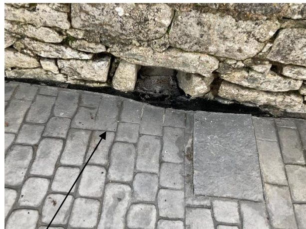
View of sealed joint at an outlet in parapet wall. General view on joint at west parapet wall.
