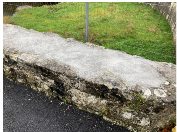
New mortar capping, upstream side, south end
