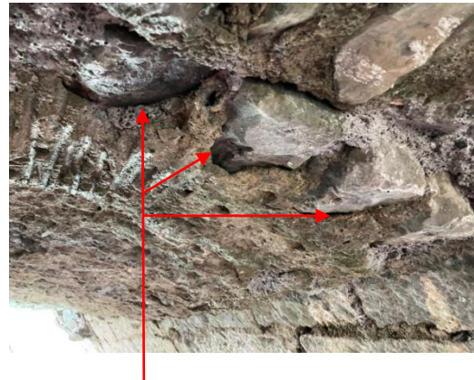
Consolidation not complete here on day of inspection
