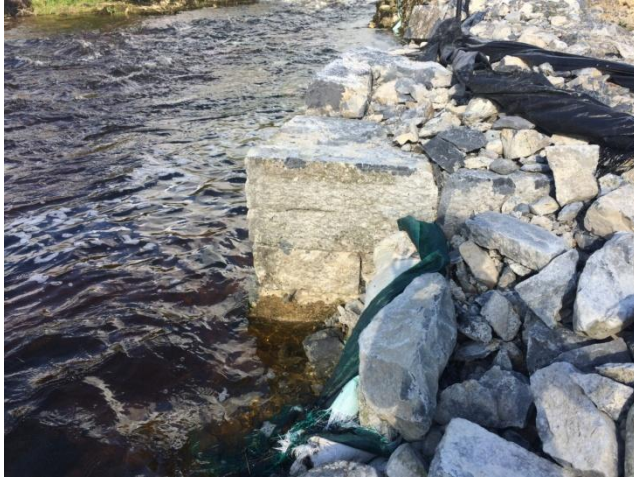
Remains of the abutment on the south side of Arch F.
