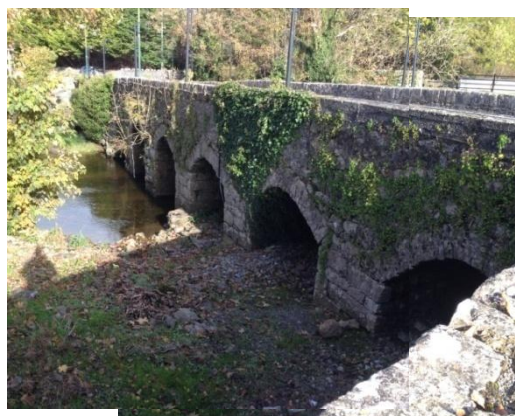
Oblique view, downstream facade.
