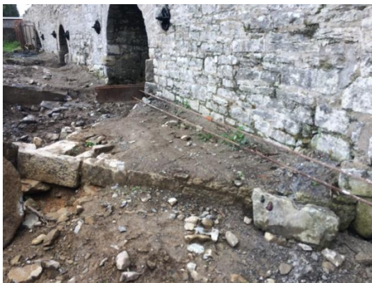
Base of cutwater between arches C and D.
