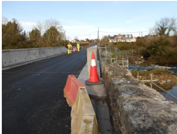
View of new bridge deck. New concrete guarding walls have to meet present day codes regarding height and strength.
