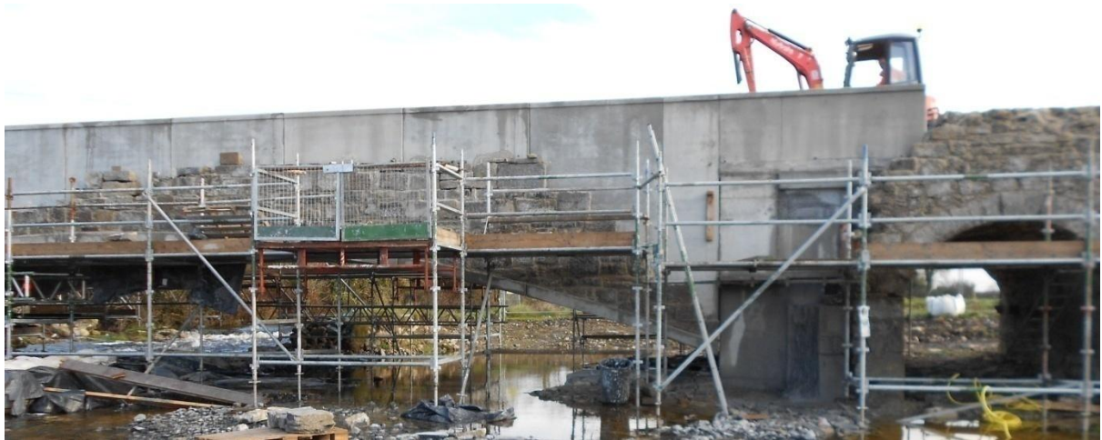
November 2019. Downstream face, concrete elements substantially complete, stone cladding progressing
