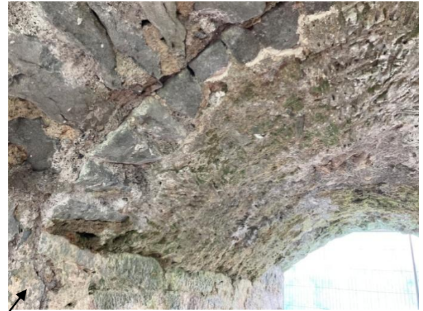
Close-up views of consolidated edges of wicker
