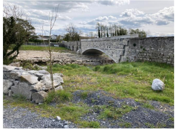
General view of upstream face from north.
