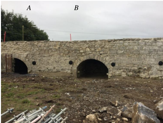
September 2019, upstream face, pattress plates and tie rods have been inserted. Stone repair and re-pointing complete
