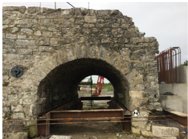
New concrete bearing under construction at south abutment of new bridge span.
