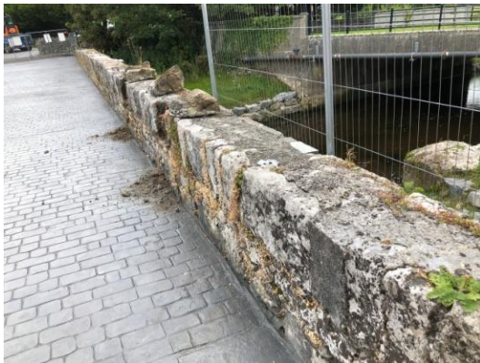
14 Sept 2020. Damaged stone and redundant light fixing. Tapping of wall to test for soundness revealed several loose stones
