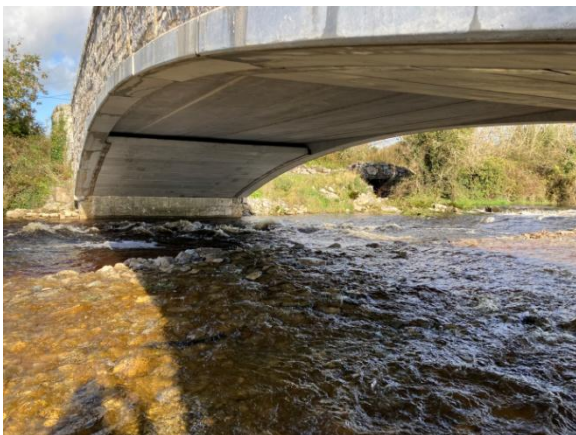
Underside view of new bridge span showing infill panels following the curve of the arch and concealing the horizontal precast beams forming the bridge deck.
