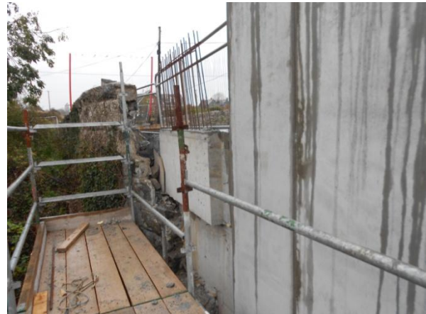
Concrete elements at the junction with the surviving stonework are cast in situ to allow careful site adjustment (north abutment)
