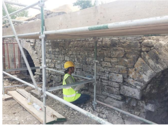
July 2019, re-pointing and raking out in progress on different parts of the upstream side of the bridge.
