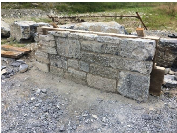
Photographs taken July 2019. Sample panels of stonework were erected for approval in preparation for building of stone cladding.
