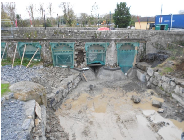
30 October 2019 general and close-up view of cutwater D/E following dismantling.
