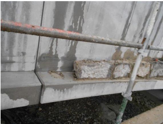
October 2019. Stone cladding commenced on the concrete 'boot' of the precast panels of the new bridge span.
