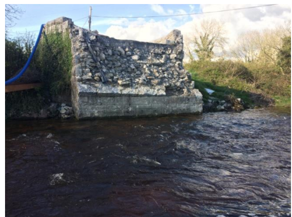
Photographs taken April 2019. Views of northern side of Arch F abutment following collapse. Note that the curved wall where the road narrowed at the bridge abutment survived. It was considered important that this example of skilled 19 th century stone craftsmanship be preserved and this was done. Suggestions of widening the bridge which would have involved the loss of this element were rejected as not in line with good conservation practice.
