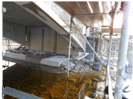
View of underside of new bridge span
