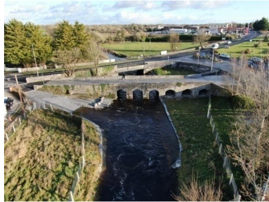
Aerial view of Craughwell Pedestrian Bridge following completion of works
