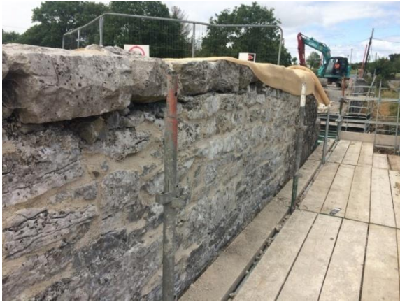
July 2019, re-pointing and raking out in progress on different parts of the upstream side of the bridge.
