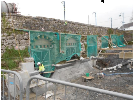
Downstream view, arches E and F in foreground. Concrete 'V' aprons are complete under arch vaults E and F and in-situ concrete aprons to base of piers to provide scour protection.
