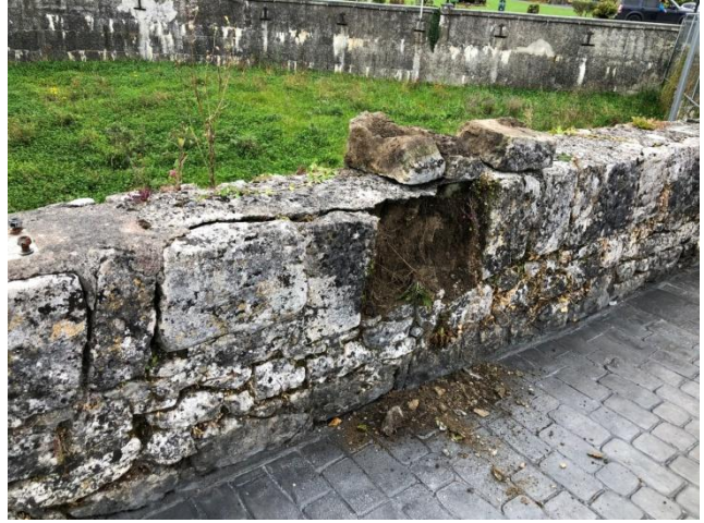
14 Sept 2020. Damaged stone and redundant light fixing. Tapping of wall to test for soundness revealed several loose stones
