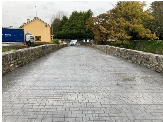
General view of repaired parapet walls
