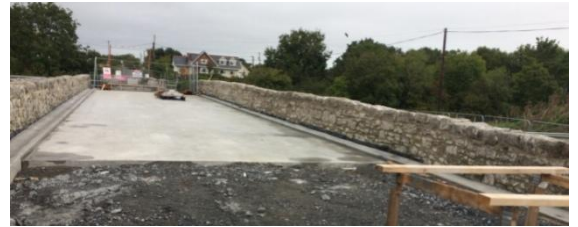
General view of repaired guarding walls at southern approach to new bridge span.
