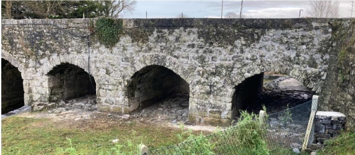
General view of re-pointed stonework above arches A, B, and C on the downstream side.
