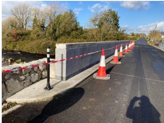
View of the bridge deck and guarding wall (looking north). Cut stone cladding was applied to the face of the concrete wall to soften its impact. Cut stone was used to clearly distinguish it from the original walls.
