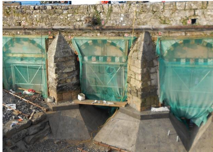
Cutwaters on 7 Nov 2019. Pointing D/E is done but not yet finished/beaten back.
