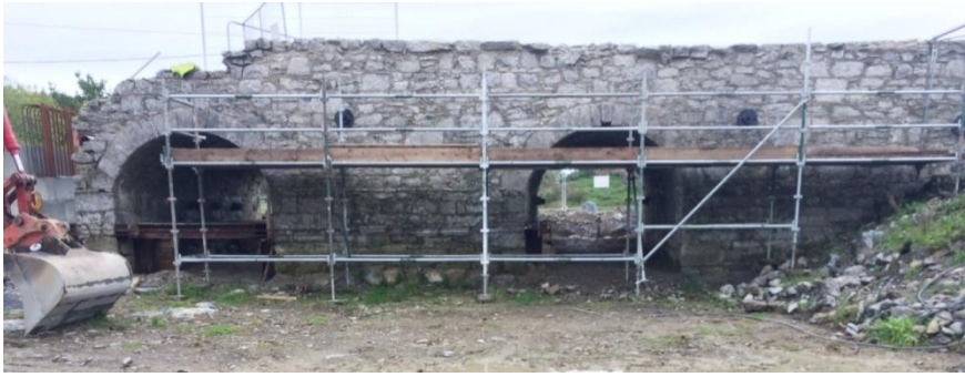
General view of downstream face, arches D and C.
