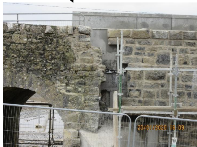
Close-up view of top of new concrete cut water and articulated break between original stonework and new stone cladding. General view of same
