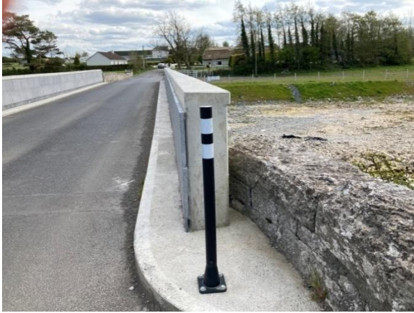
Other view of north-west junction where curved wall meets new guarding wall
