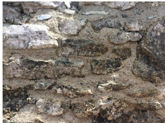
Sample panel of re-pointing for approval. Texture of mortar is in keeping with original. Washed chip was added to the sand.
