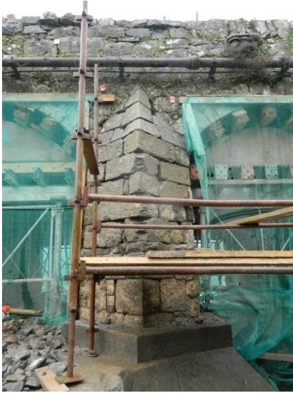
Cutwaters on 7 Nov 2019. Pointing D/E is done but not yet finished/beaten back.
