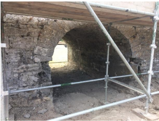
July 2019, re-pointing and raking out in progress on different parts of the upstream side of the bridge.
