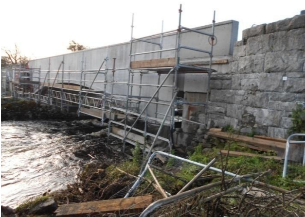
Stone cladding not commenced on upstream side. Note that the original curved stone wall at this north abutment is well preserved.
