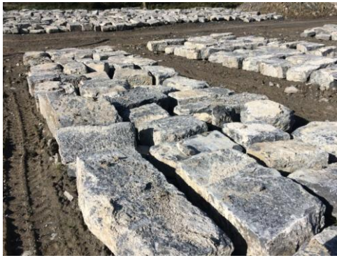
Photographs taken April 2019. Comprehensive careful sorting of stone was undertaken following the collapse.
