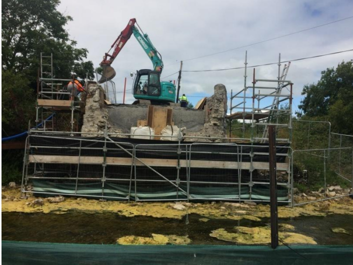
July 2019, preparatory work underway for new concrete support at northern abutment.
