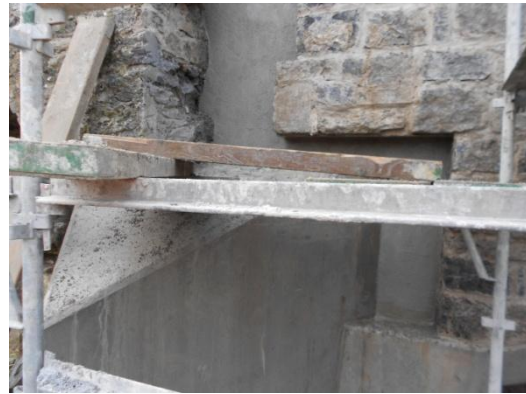
January 2020, stone cladding on the sides of the new bridge is close to completion Upstream side looking north
