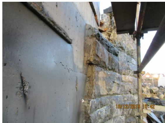
Stone cladding not commenced on upstream side. Note that the original curved stone wall at this north abutment is well preserved.
