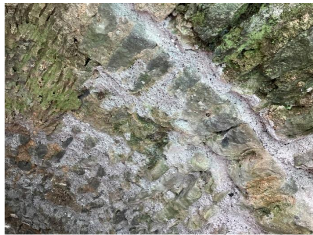
View looking upstream General consolidation of vault stonework using pinnings and coarse mortar mix.
