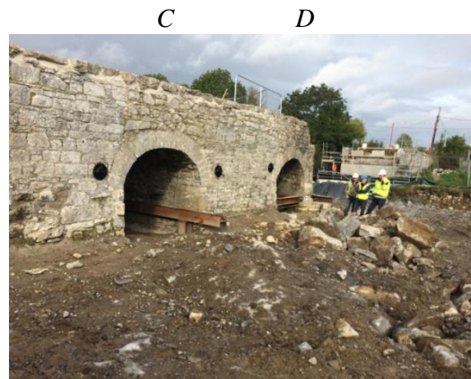
September 2019, upstream face, pattress plates and tie rods have been inserted. Stone repair and re-pointing complete
