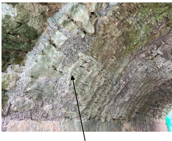
Looking upstream, consolidation of wicker edges and general consolidation of stonework
