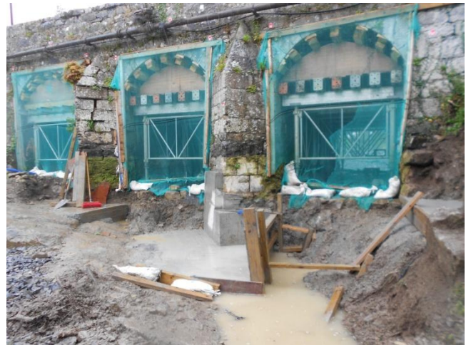
27 August 2019, cut waters prior to consolidation works.
