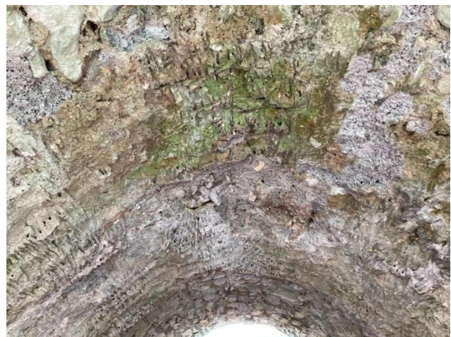
Looking upstream, consolidation of wicker edges and general consolidation of stonework
