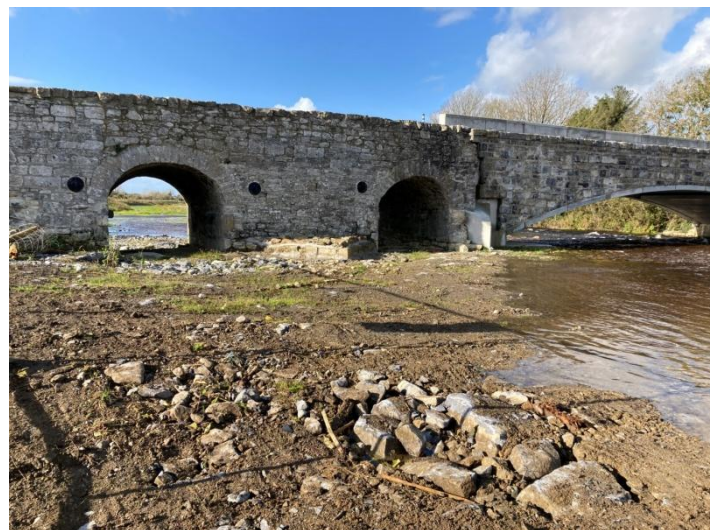
Upstream view from south with new concrete cutwater at arch D in foreground
