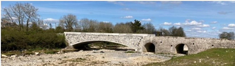
General view of downstream face from south
