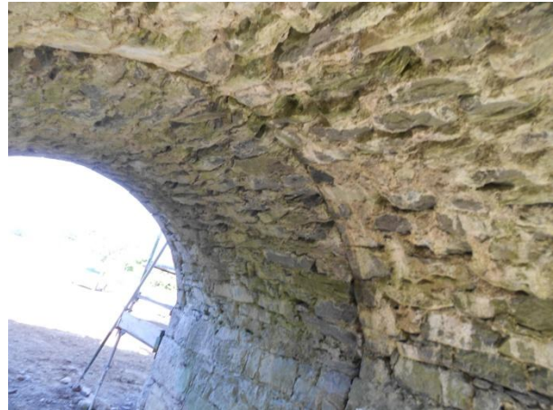
Photographs taken 10 August 2018 Accumulated material on arch floor being removed. Joint between earlier and later construction clearly visible on underside of the vault.
