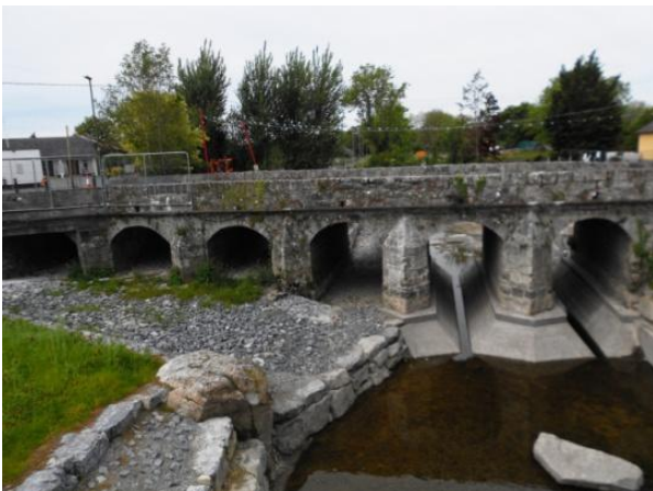
May 2020 prior to removal of upstream dam.
