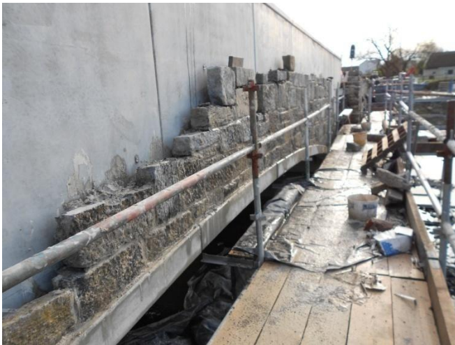
November 2019. Downstream face, concrete elements substantially complete, stone cladding progressing
