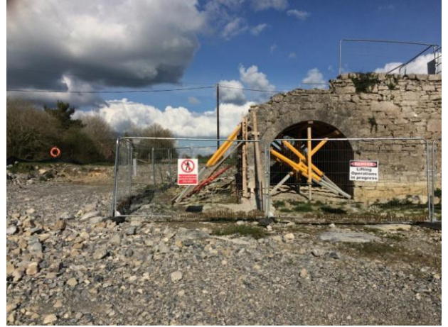
Arch D is shored after the collapse.
