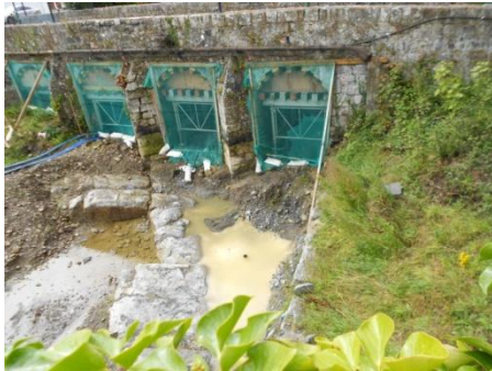
27 Aug 19. Note positioning of large boulders in river bed as part of OPW strategy for water management
