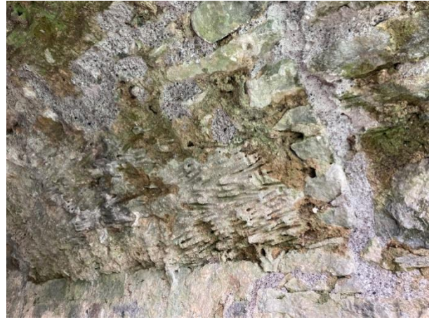
Further views looking upstream. Some loss of wicker noted on this side compared to extent recorded in April 2019
