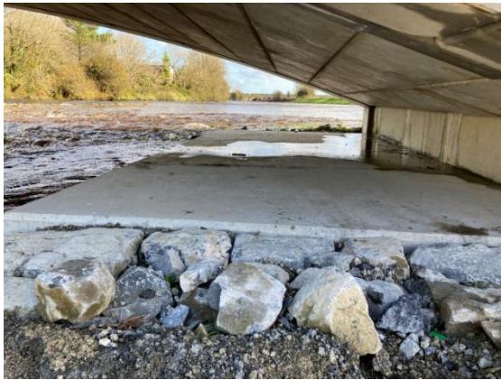
View under the new bridge span looking upstream.
