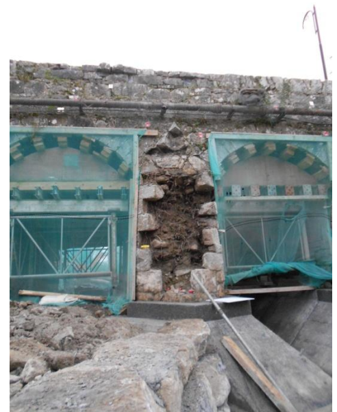
30 October 2019 general and close-up view of cutwater D/E following dismantling.
