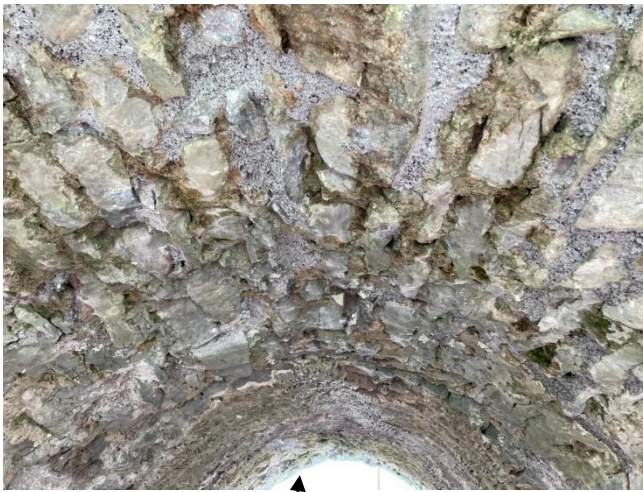
Looking downstream. ↑ General consolidation of vault seen in foreground.
