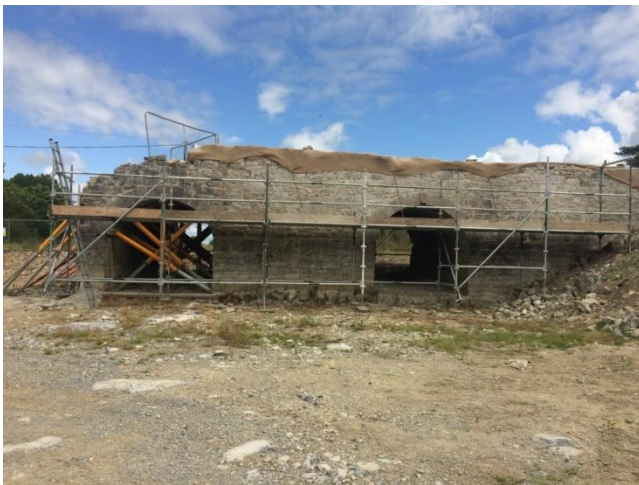
Re-pointing and patch repair well progressed on downstream face of bridge.
