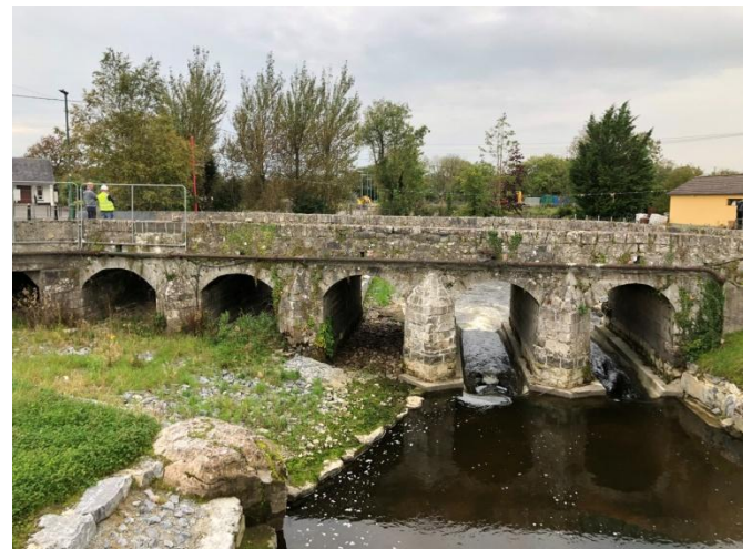
June 2020 when dam was dismantled and river restored to its primary channel. Bypass channel remains open to take water in the event of flood.
