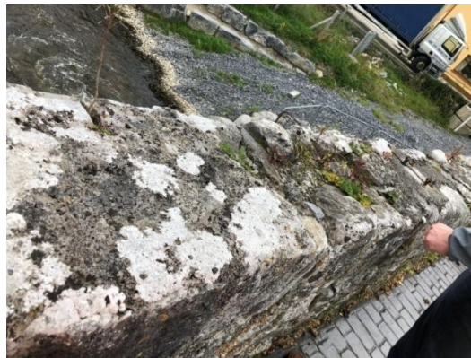
Capping in poor condition
