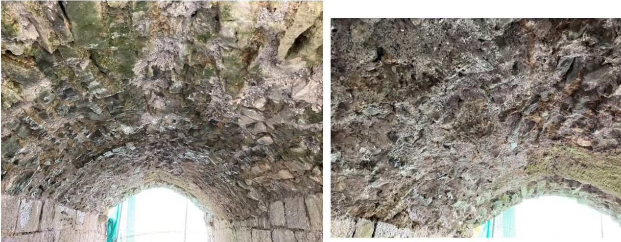
Views looking downstream, Arch A, post works.
