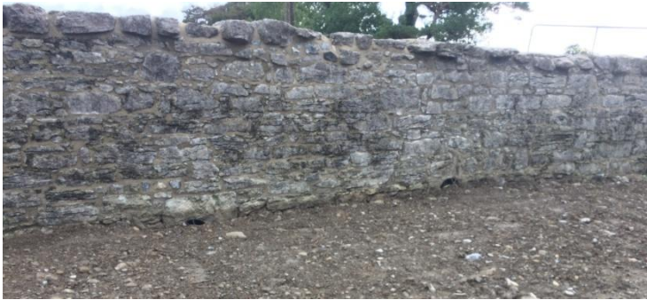
View of repaired guarding wall, downstream face.
