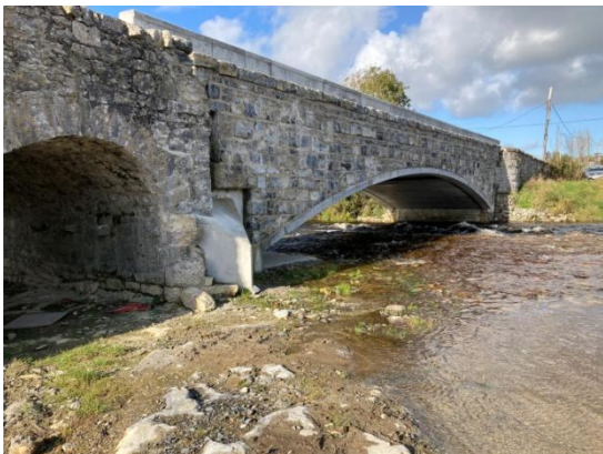
Upstream view from south with new concrete cutwater at arch D in foreground
