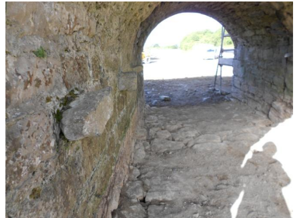
The collapse of the bridge arches at Dunkellin occurred on 22 Aug 2018.
