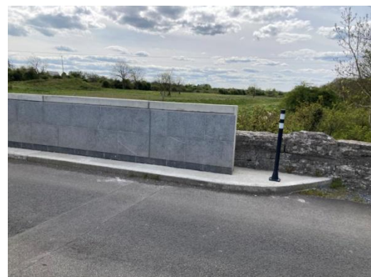
View of north-west junction
