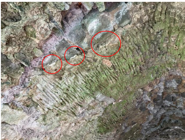
View looking upstream Fine mortar mix was injected behind the wicker centring to re-adhere it to the background stonework. New mortar is just visible at the edge of the wicker (circled red)
