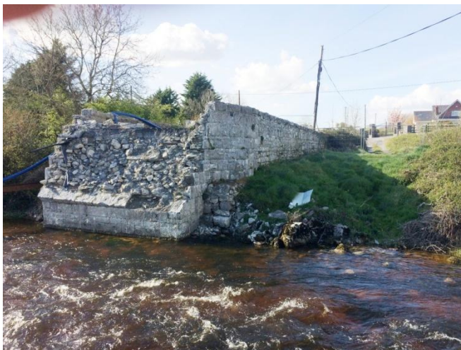
Photographs taken April 2019. Views of northern side of Arch F abutment following collapse. Note that the curved wall where the road narrowed at the bridge abutment survived. It was considered important that this example of skilled 19 th century stone craftsmanship be preserved and this was done. Suggestions of widening the bridge which would have involved the loss of this element were rejected as not in line with good conservation practice.
